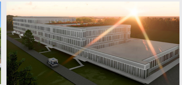
Example of a Land-based 4-Floors Main Hospital of up to 82,000 m 2 (882,640 ft 2 ). Designed for comprehensive specialist care.
